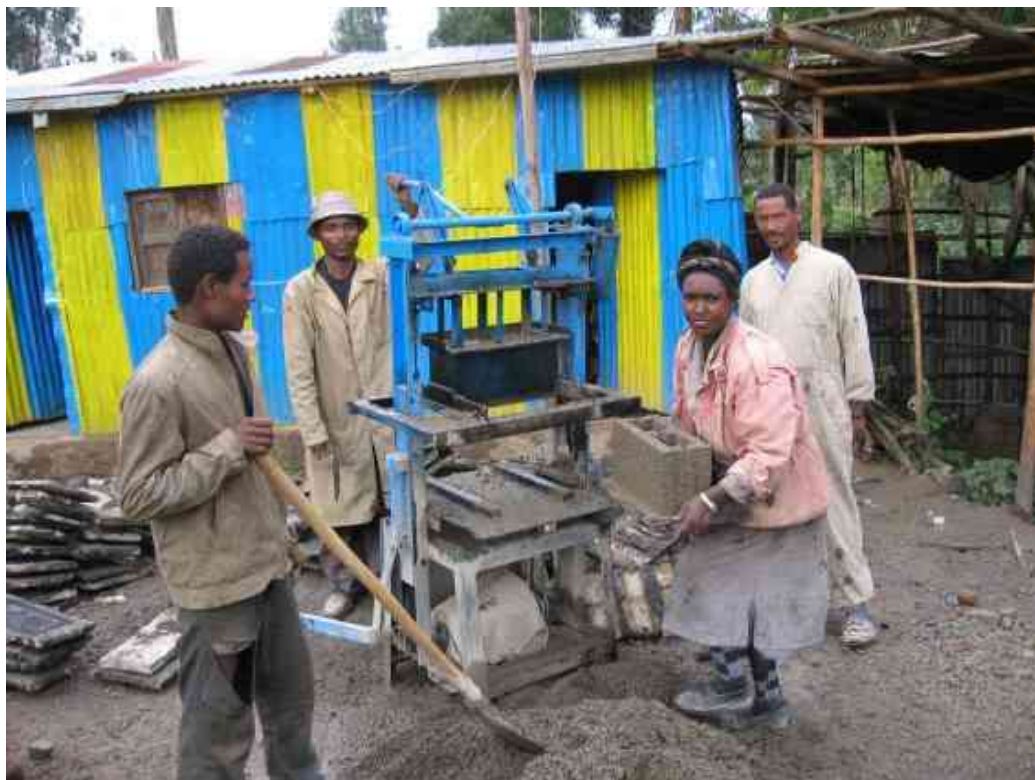
Production of hollow-blocs
