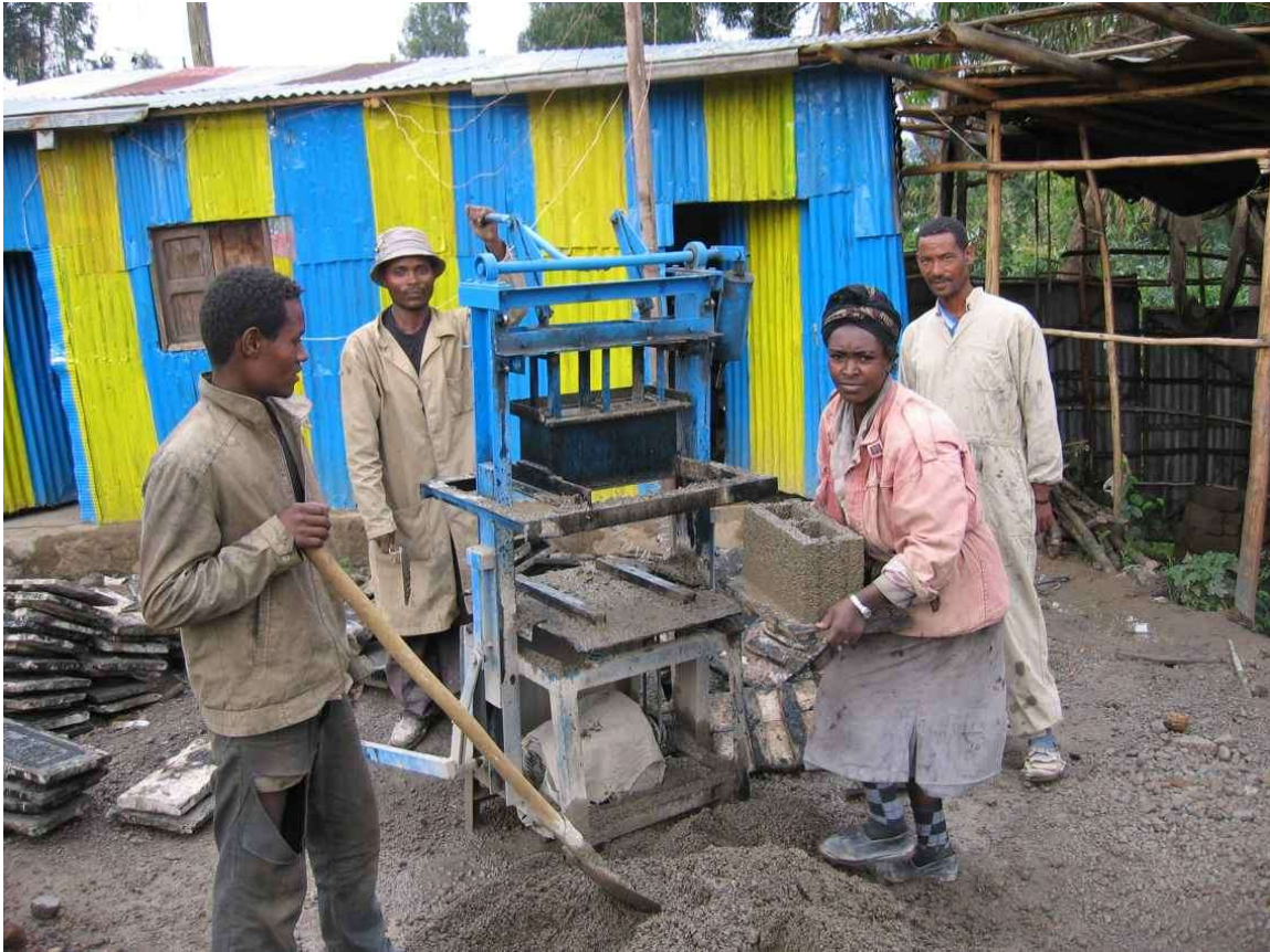
Dawit Ejigou, Production of hollow-blocs, Addis Ababa
